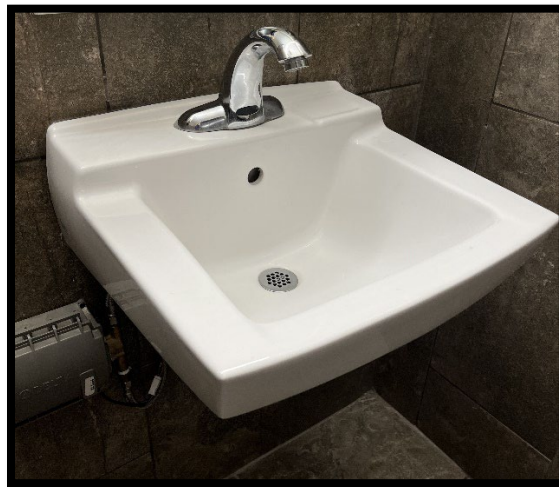
Figure 3: New Sensor Faucet Installation at Arena
